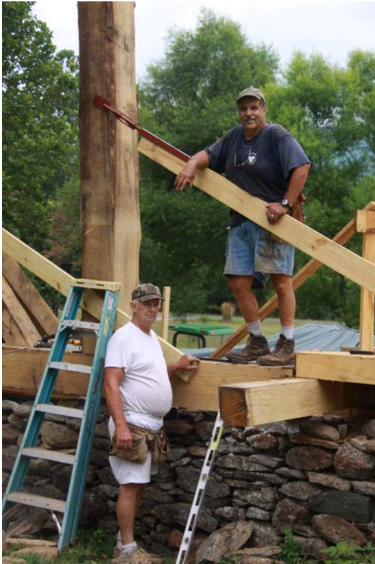
Restoration of Graves Grist Mill
